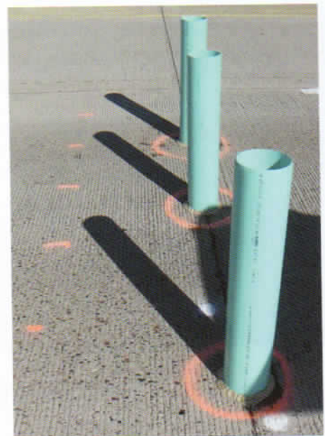
Joint Infiltration testing was conducted on in-service pavements
