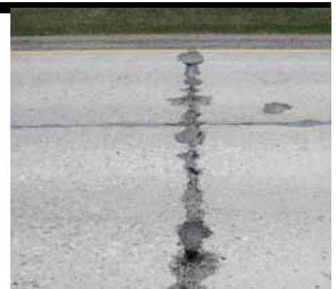
*High severity spalling at transverse joints - sections of the project with spalling this severe at each joint were removed and replaced.*
