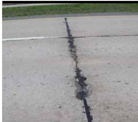
*Spalling at transverse joint - location to be repaired with partial depth repair techniques.*
