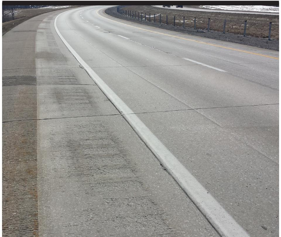
lion. The expected pavement life extension for ground pavement is 10 to 15 years. The average cost of diamond grinding during this five year period was \$2.75 per square yard.
