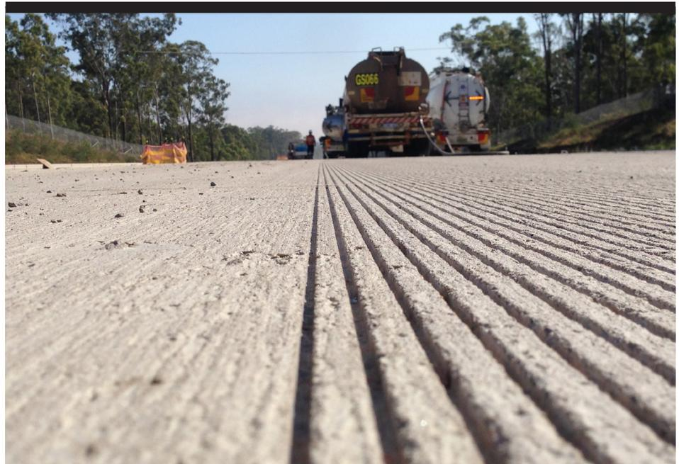
ly used on existing concrete pavement in NSW since 2009 to reduce pavement roughness and increase skid resistance, but the noise attenuation provided by conventional diamond grinding was similar to that of dense-graded asphalt.
