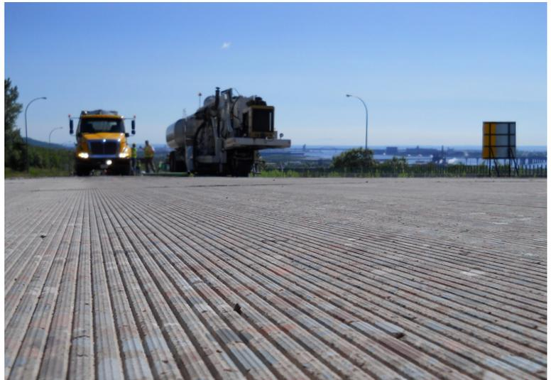
in a lower overall noise level, while the grooves, which provide significant macrotexture, increase the resistance to hydroplaning by moving water out of the tire contact patch area. The NGCS surface can be constructed on new roadways or existing roadways.
