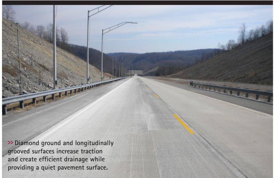
>> Diamond ground and longitudinally grooved surfaces increase traction and create efficient drainage while providing a quiet pavement surface.
