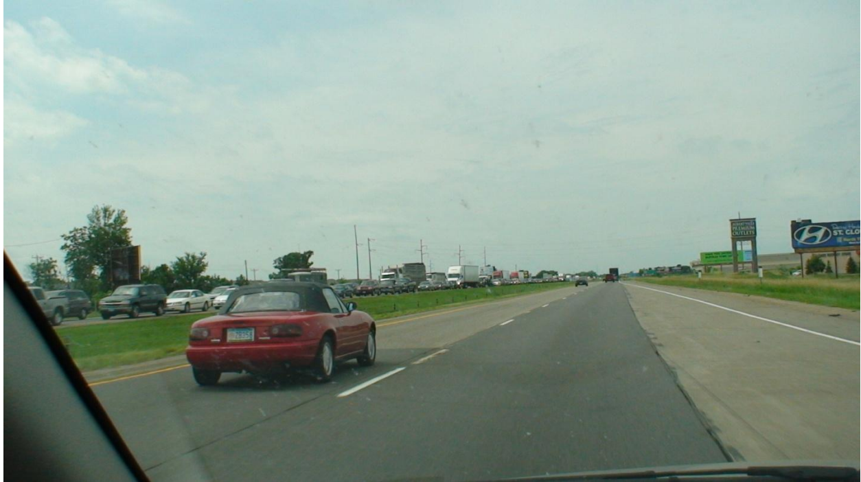
Figure 3 Photo of I-94 EB Traffic Backup Resulting from Construction Project to the East
