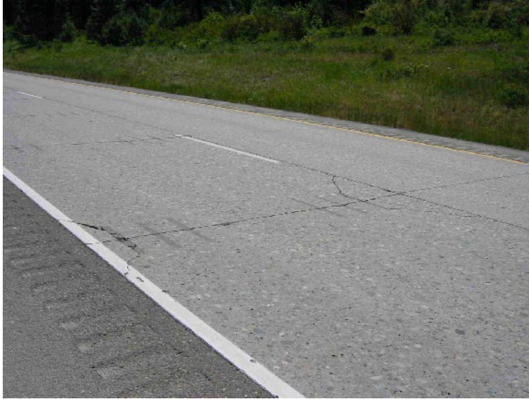
FIGURE 7 45-degree cracking.
