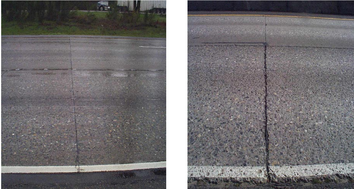
FIGURE 9(a) and (b) Surface texture for diamond grinding and roto-milling.
