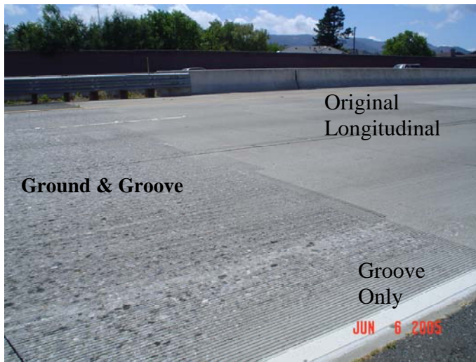
Fig. 5: Photograph of textured section of SCL 85 indicating both grooving and grinding and original
