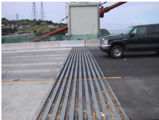
Fig. 12: Photograph of expansion joint on the new span of the Carquinez Bridge – AC bridge to the right, transversely tined PCC viaduct surface to the left
