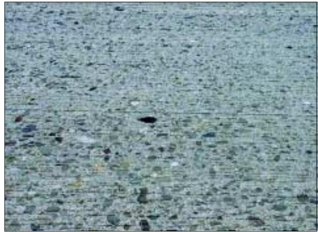
Figure 2. Route 101 surface after diamond grinding.
