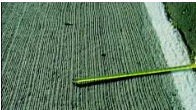
Figure 1. Longitudinal grooves of Route 101 at the test segment.
